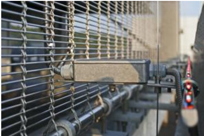
Picture 6: The stainless steel wire mesh is illuminated indirectly by the LED-tubes.
